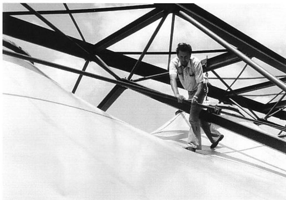
Checking of the finished membrane structure
