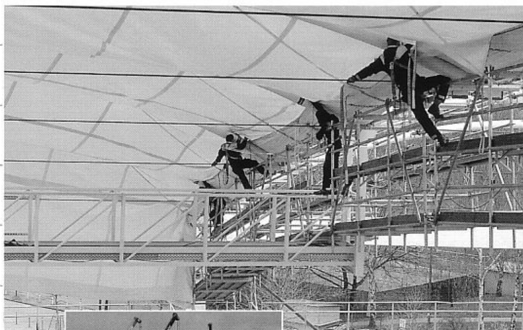
Erection of the prefabricated membranes
