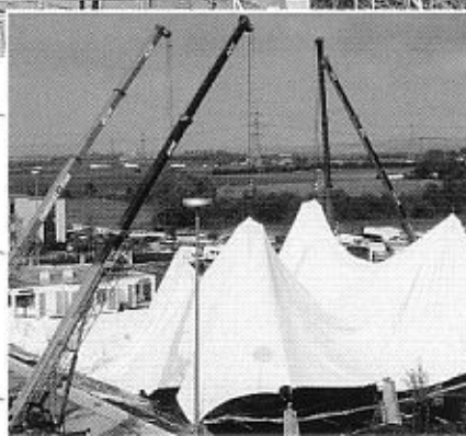
Erection of large membrane elements
